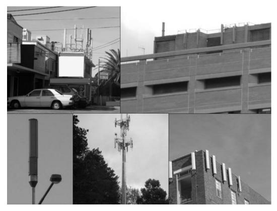
Figure 1—Mobile phone base stations ("antennae" or "masts") in Australia. Upper left: Community shop roof showing plethora of flat panel antennae. Upper right: Hospital roof with flat panel antennae painted to blend in. Lower left: Top of a street light pole. Lower center: Mast erected next to a daycare center. Lower right: Antennae mounted on an office block top floor.
